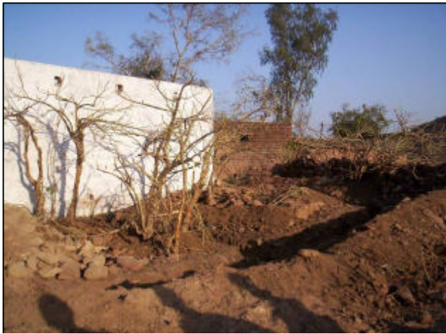
Foundation for the labour room behind the ayurvedic dispensary
